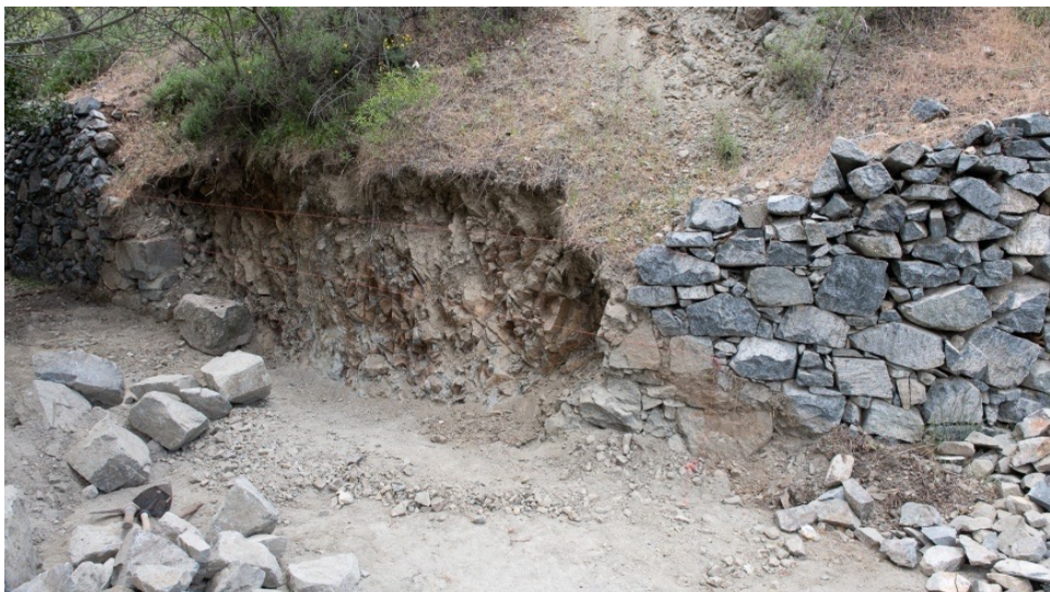
Wall A before
